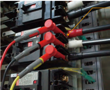
Magnetic design (diameter: 11 mm)
