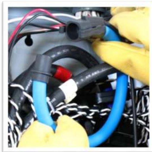
Photo 2: Install CT Around Conductor.
