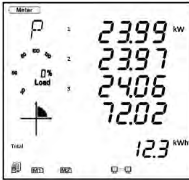
Figure 3-7 - Three-Phase Power Page
