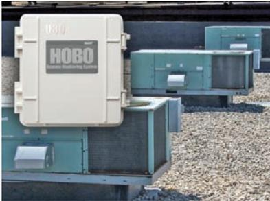
Web-based systems enable real-time, remote access to your data via cellular, Wi-Fi, or Ethernet communications. They can be configured with any combination of external smart sensors, and have been designed with an industrial-grade, tamper-proof enclosure. This enables them to be used in indoor HVAC monitoring projects, as well as outdoor projects such as rooftop HVAC system monitoring.
